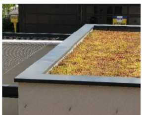
Toiture extensive (substrat 6cm)
