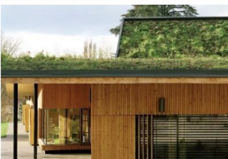
Toiture intensive (substrat 12 cm)
