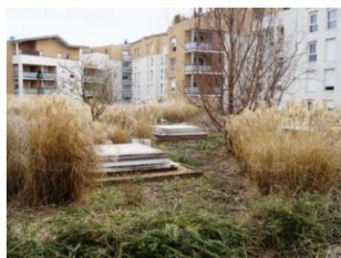
Toiture intensive (substrat 50 cm)
